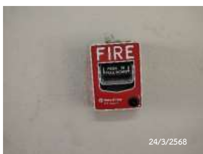
Fire Alarm Manual Station
