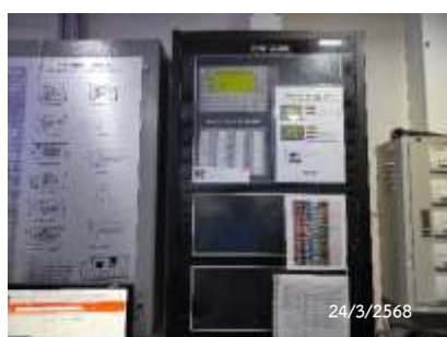
Fire Alarm Control Panel
